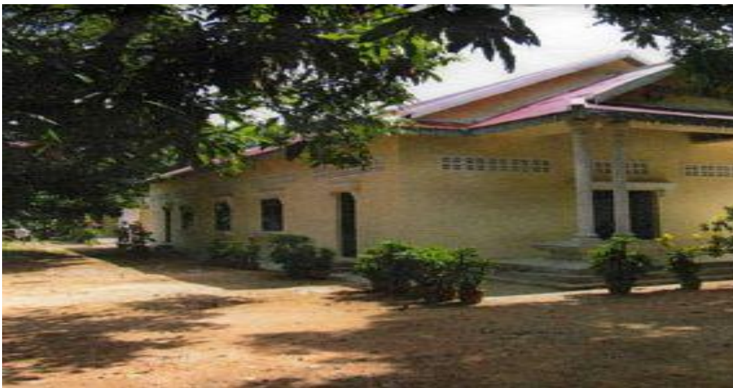
Church in Seung, Cambodia, built by a team from Dover Baptist Church, working with Missions Door and Cambodian Ministries for Christ
